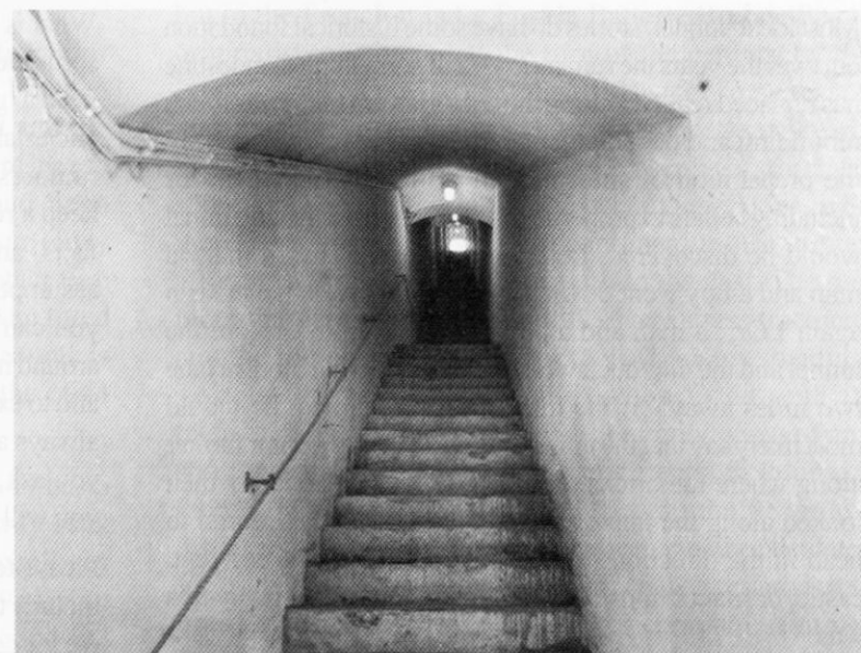
Looking up the steps towards Roedean School
